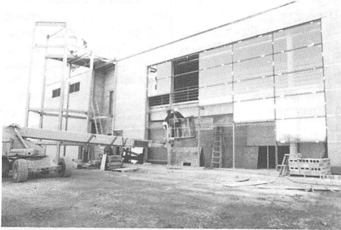
PETTIT NATIONAL ICE CENTER The entrance was starting to take shape.
