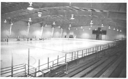
A clear span building enclosing a 100x200 ice surface.
